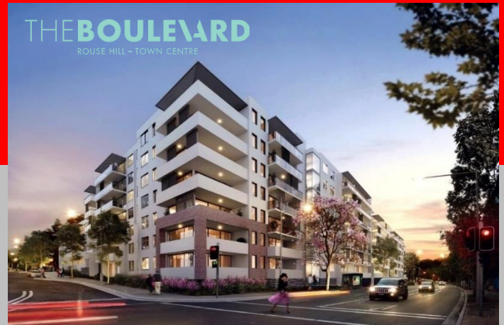
THE BOULEVARD – ROUSE HILL TOWN CENTRE
