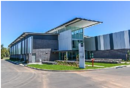
The new Tamworth Education Centre
