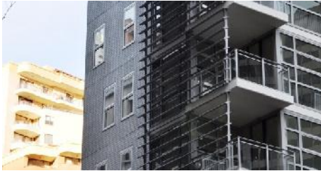
The Jade Apartments on Sussex Street
