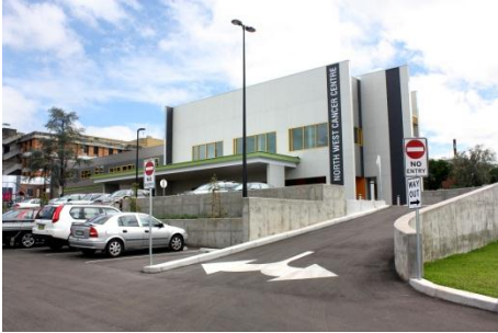
The new extension to the Tamworth Hospital
