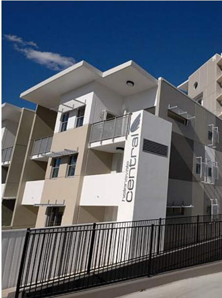
'Central' residential apartments, Helensvale
