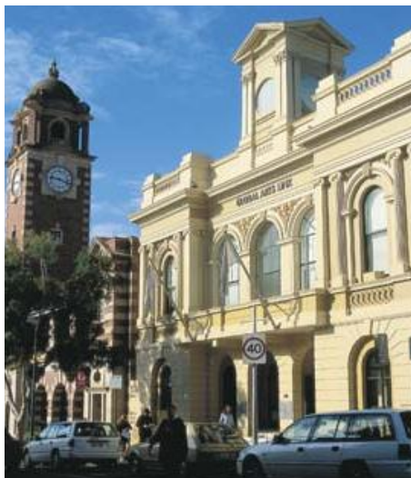
Ipswich Clock Tower Landmark
