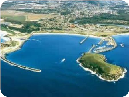
Coffs Harbour Jetty
